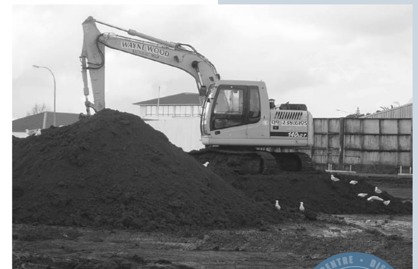
Local subcontractor Wayne Wood has begun earthworks at the site.
